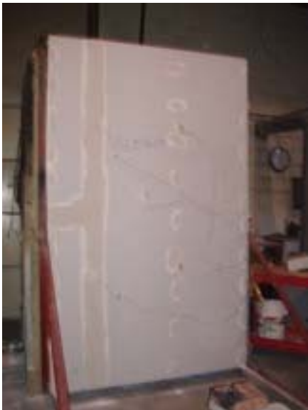
Completed unexposed side
