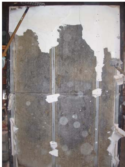
After test: showing back of unexposed side
