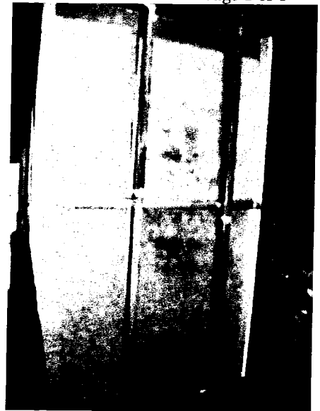
5/8" SCX gypsum wallboard placed on exposed side
